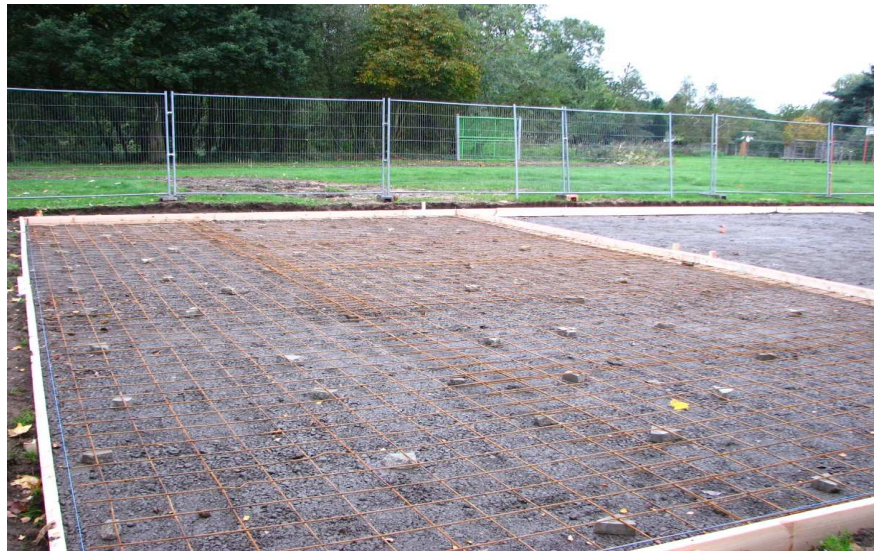
Photograph B – Steel reinforcement for the base (28 th October 2006)
