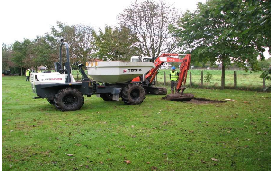
Photograph A – Excavation work gets underway (4 th October 2006)
