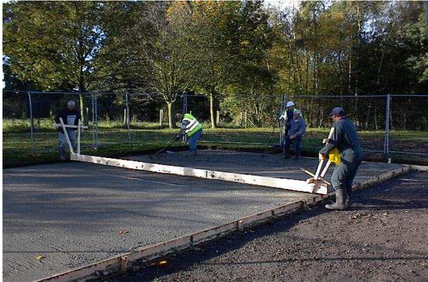
Photograph C – Laying the concrete base (November 2006)
